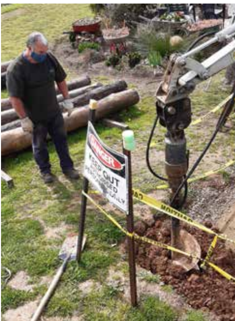
(l to r): Excavating the footings; cutting the poles; installing beams, rafters and strapping
