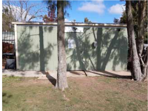
The original shed before the shelter was built
