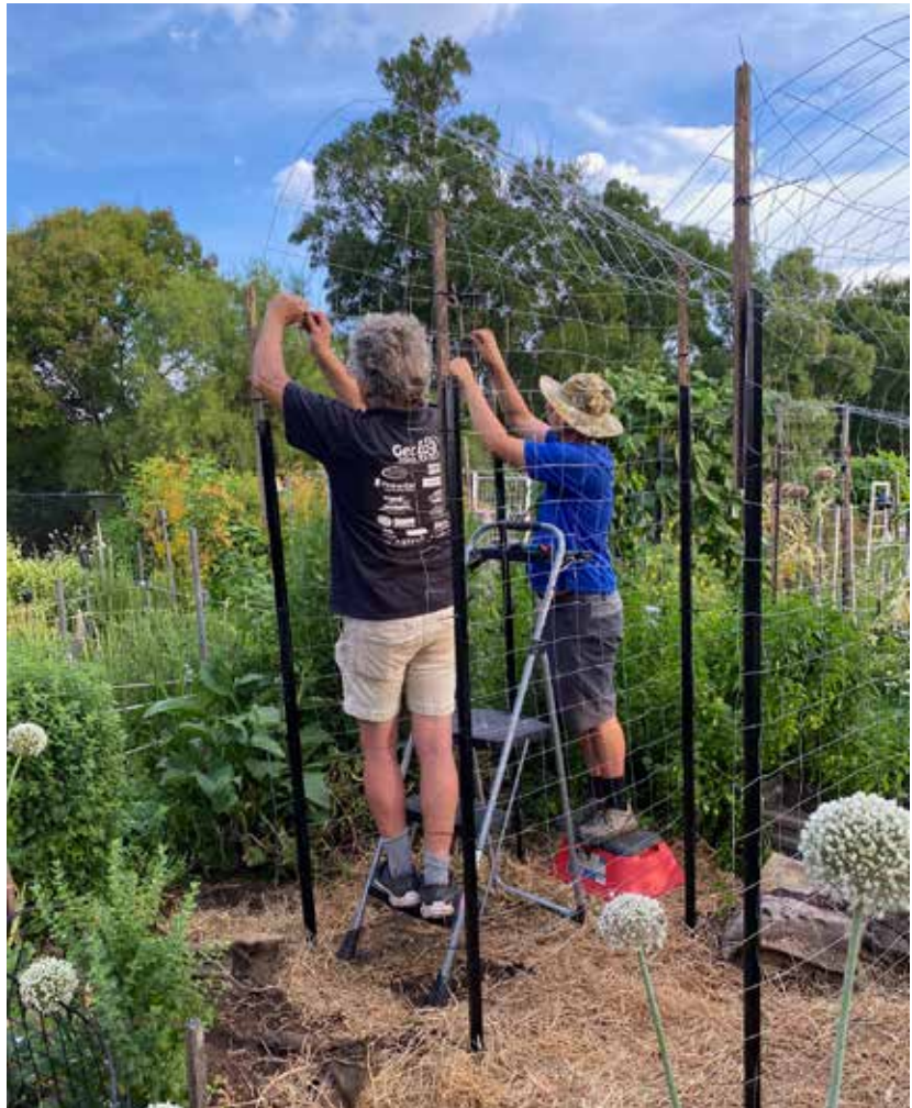
Peter and Markus, resident engineers, building a new trellis. Photo: Didi Sommer.
