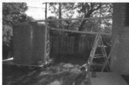
Left: Protank—my professional but DIY installed tank (Option 1). Far Right: Drums on crate—overflow tanks for dipping the watering can into (Option 2). Centre: Drum under a shed gutter.
