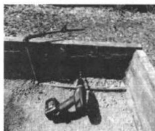
Drain holes drilled at 100mm
