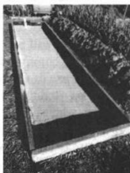
Laying in 100mm of washed sand
